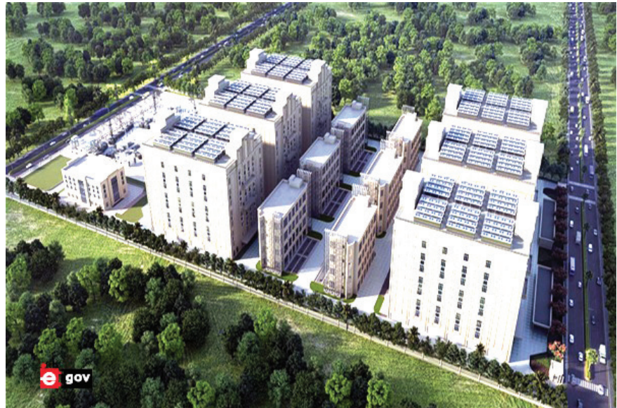
Upcoming Data Centre Park in Greater Noida, UP
